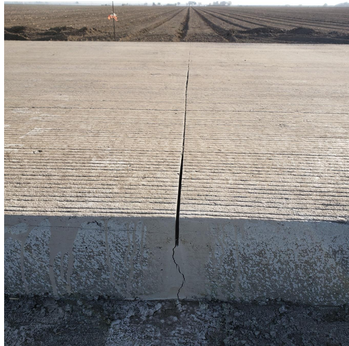
Sawcutting at 1/3 depth
