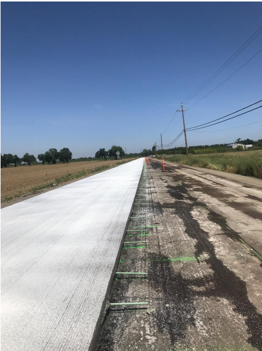
Standard curing compound at standard rate
